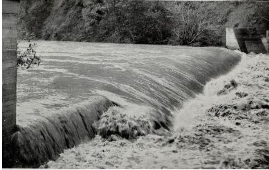
The dam to impede the flow of water down Niles Canyon about one mile south of the Sunol Water Temple.
